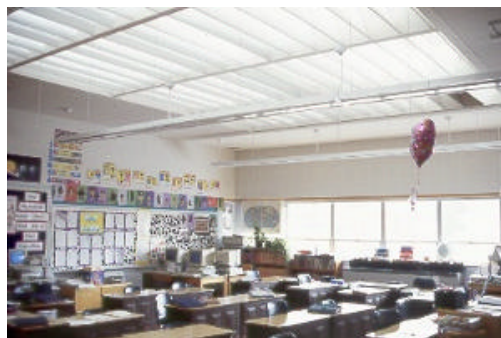
Central Skylight and Diffusing Louvers
